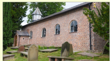
St John's church recently re-pointed
